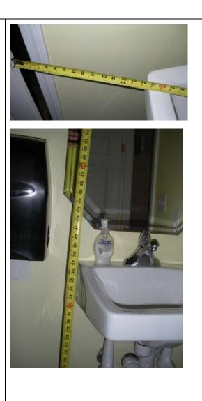
Reposition the grab bars by moving 6" forward. Bar should be 12" max from back wall and extend 54" from back wall.
