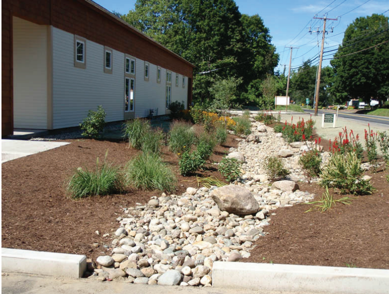
A rain garden along Route 9 in Hadley, captures storm flow from a drive and parking lot. This photo is taken just after installation and before plants are really established.
